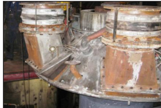
Top section protected internally with ARC being lowered into place
